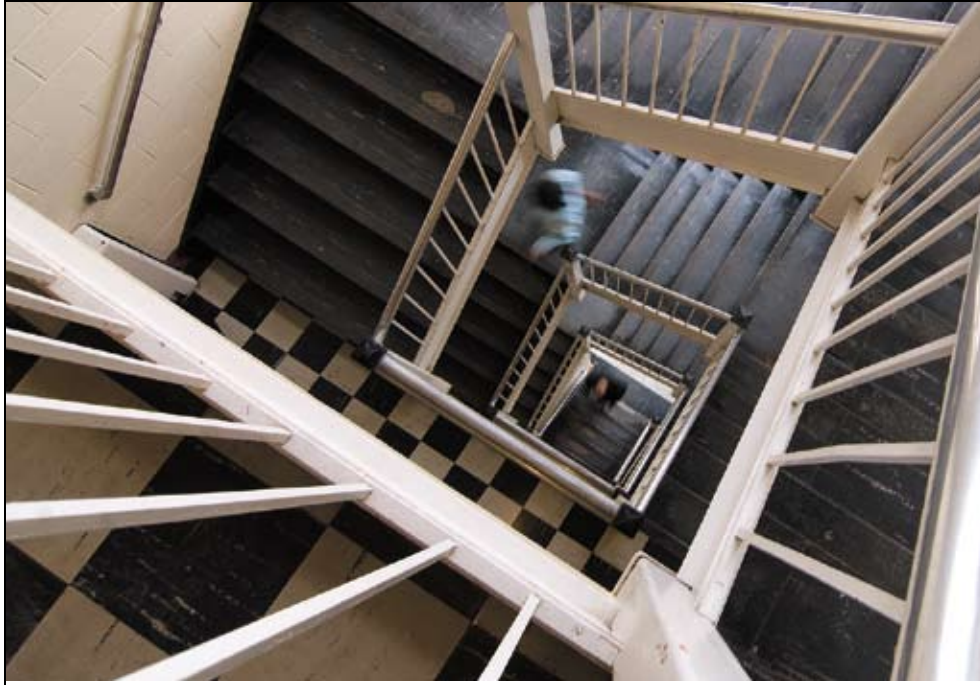
A stairwell in Gentry Building.
